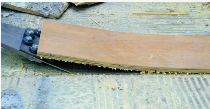
Removal of pressies
