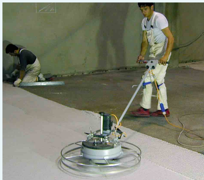
The extra long guide handle is infinitely adjustable to the height of each individual operator. The radius of action is large thanks to a tool diameter of 820 mm.
